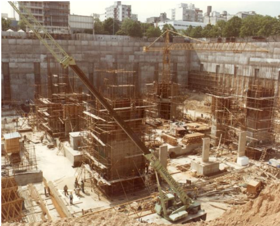
Figure 1: Excavation during the construction of the complex
