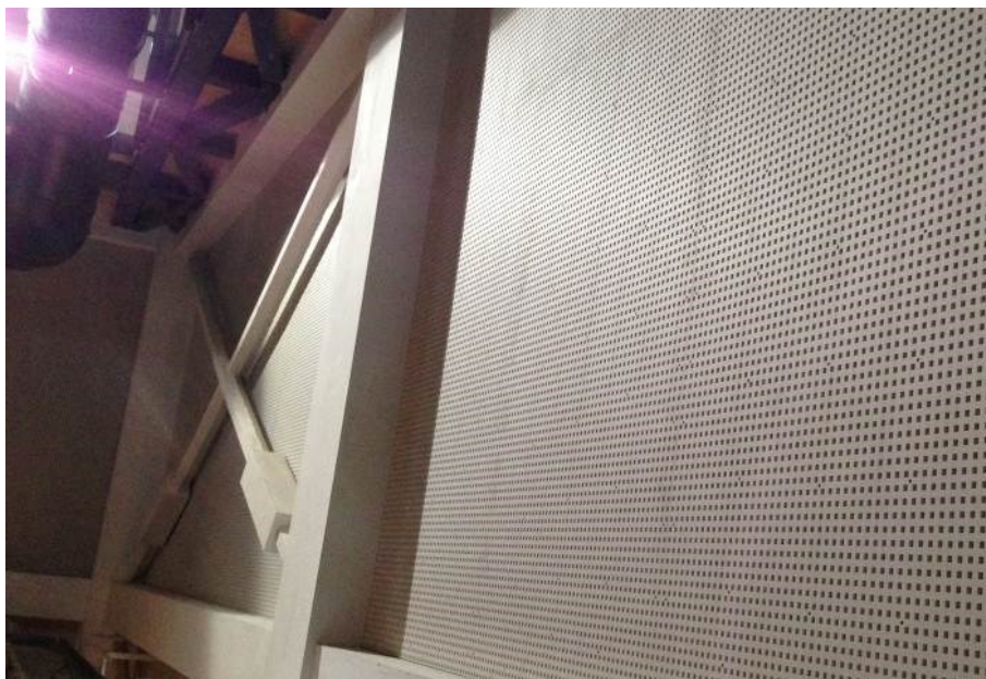
Figure 3: Materials for a simple and effective treatment of the stagehouse. The design needs to be developed numerically in the context of the coupling of stagehouse and main hall.
