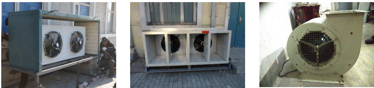
Figure 1: The most commonly used cooling fans in the station
